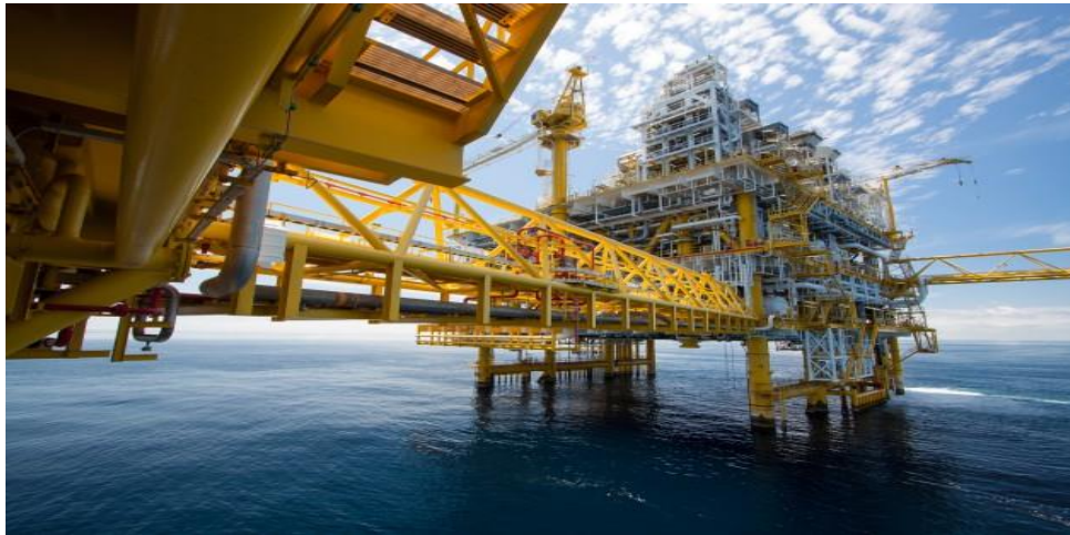
شکل ۴- Fixed Jacketed Structure
